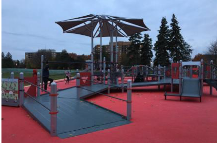
Double-wide ramps allow for wheelchairs to roll side-by-side and give enough room to change direction.
